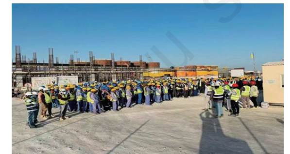
Oil tank project -UAE
